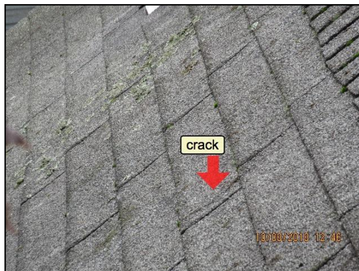
10. Left Side Crack, Stone loss, Worn
