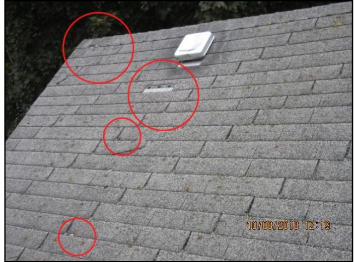
3. Right Side Damaged/Missing Shingles
