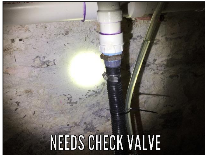
88. Missing check valve
