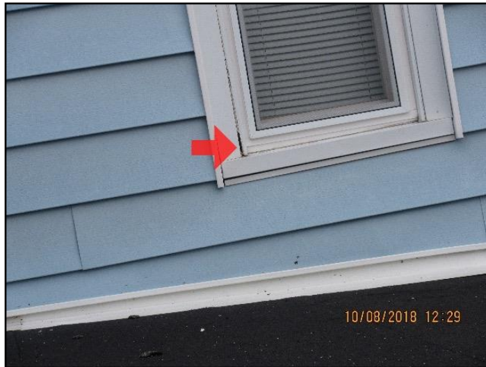
24. Paint and Caulking - deteriorated / missing
