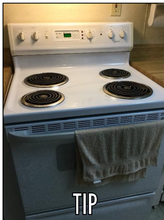
104. Anti-tip device missing
