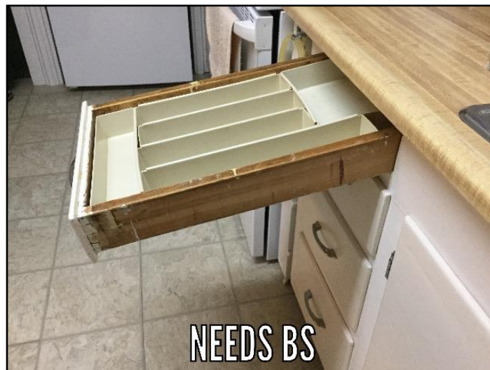
96. Drawers - missing or defective stops
