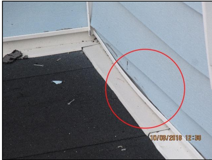
16. Damage, loose, open seams, patched
