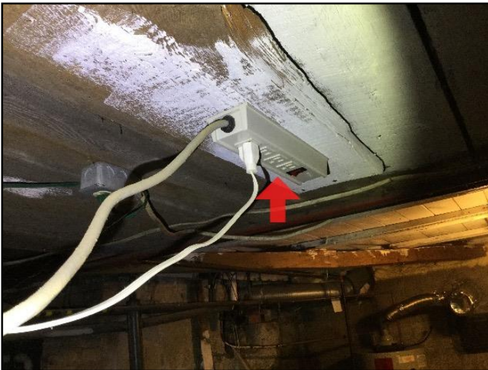
61. Extension cord used as permanent wiring
