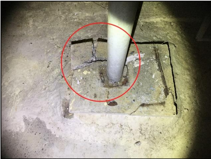
37. Damaged Pier
