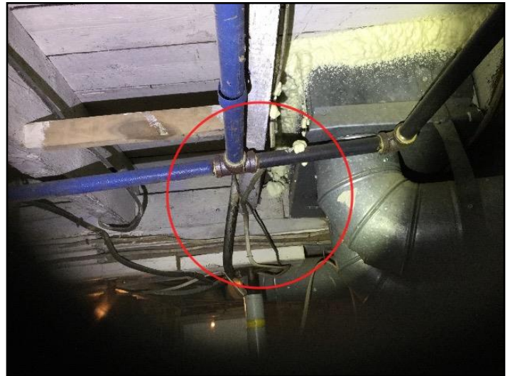
48. No blocking, bracing or bridging
