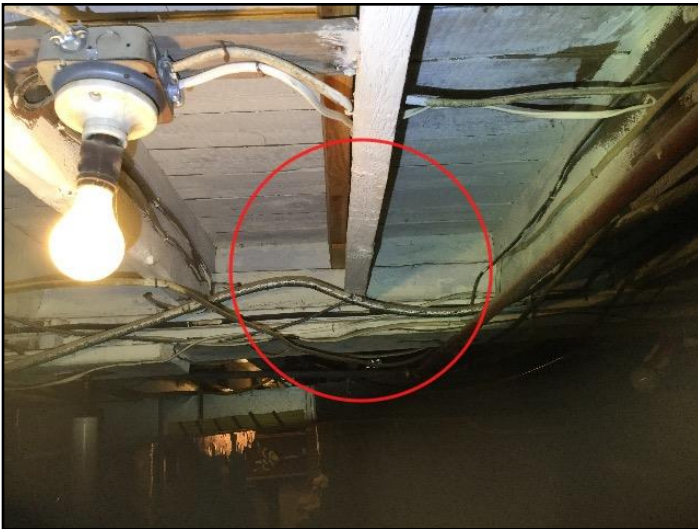
47. No blocking, bracing or bridging
